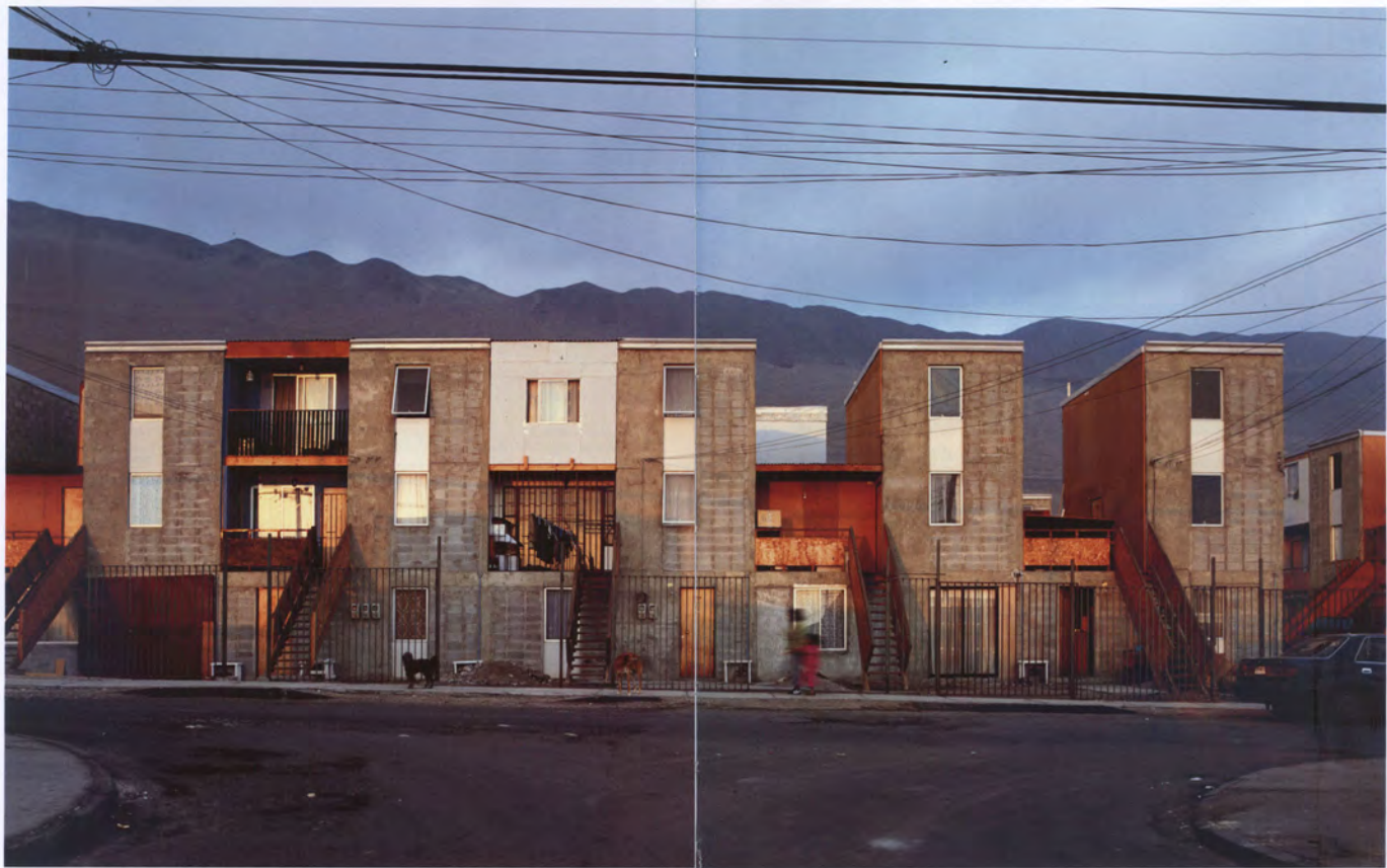
Fig. 5: General view of the facade with addition, June 2006.
