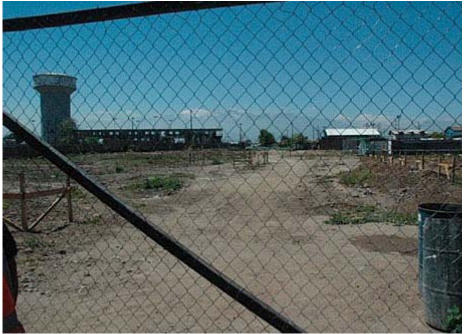
The site of the second phase of the ELEMENTAL development in Lo E where a shantytown once stood. Even from Santiago's most impoverished neighborhoods, the majestic Andes are visible in the distance.
